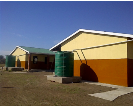
Above is the project installation of new Jojo and tank stand base construction of new ablution blocks
