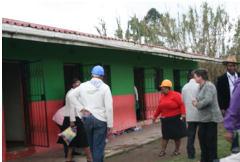
Ugu District Officials preparing to start painting
