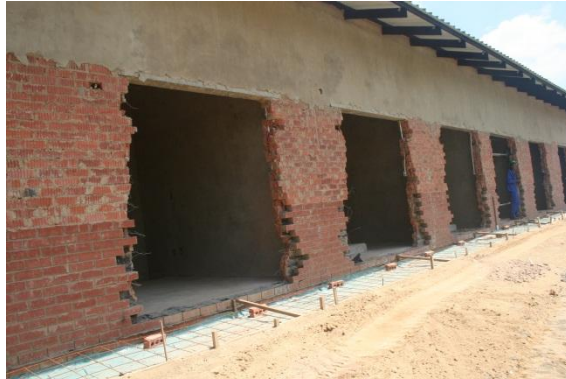
The New CSSD and theatre currently under construction
