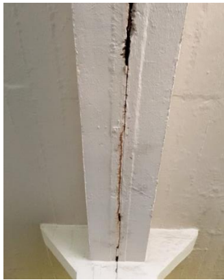
Picture 5: Water leaks through structural joints on soffit from floor above
