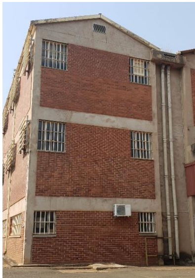
Picture 1 External façade and Rain water goods requires maintenance
