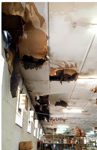
Picture 8: Roof and ceiling damage
