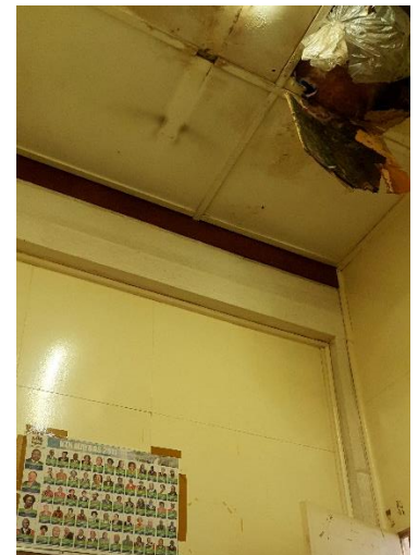
Picture 10: Roof Damage to Store Office on First Floor
