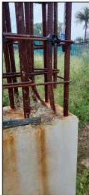
Showing excessively cranked and corroded reinforcement.
