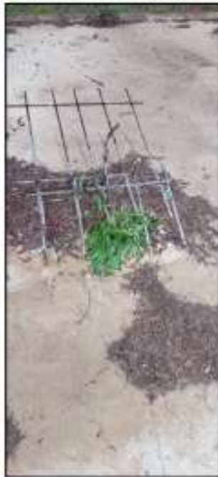
Showing staircase starter bars.
