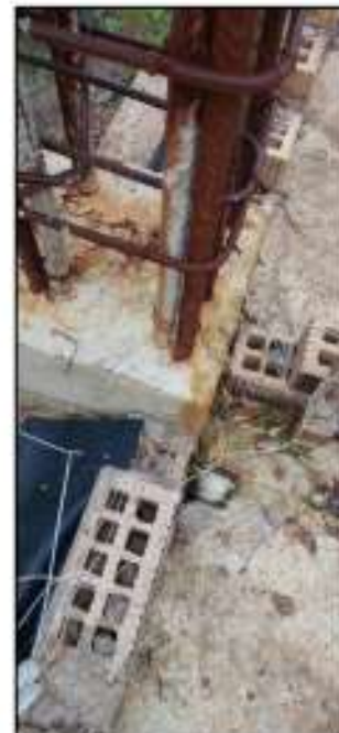
Showing insufficient cover to reinforcement.
