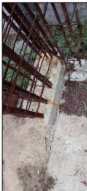
Showing insufficient cover to reinforcement and on-site not approved cranked bars.
