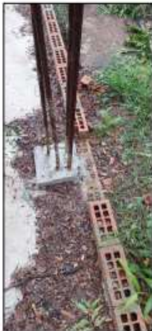
Showing insufficient cover to reinforcement & bent bars.
