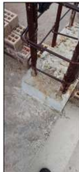
Showing spalling of concrete and subsequent cracking.
