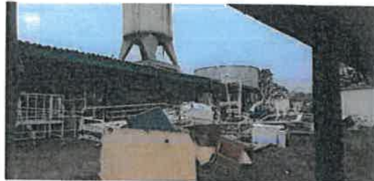
Image 10 Exterior condition of SCM building (Source: Author)
