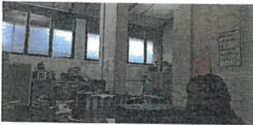
Image 7 Interior condition open plan offices of SCM building (Source: Author)
