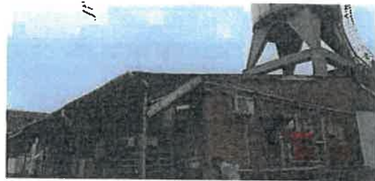
Image 8- Exterior condition of SCM building (Source: Author)
